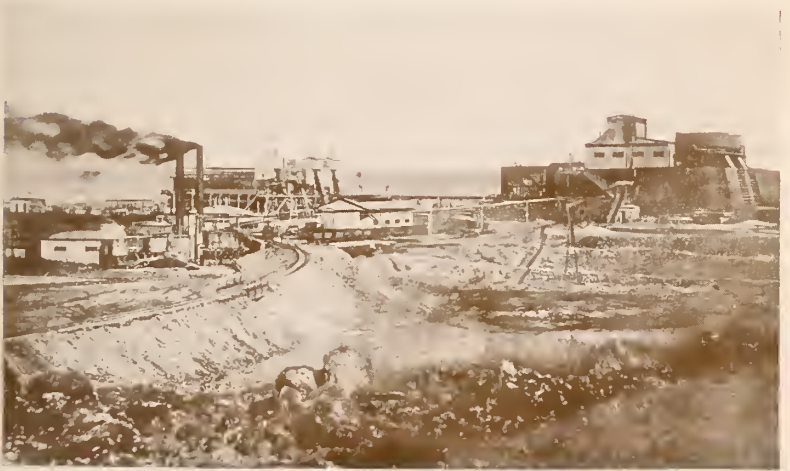
General View of Nitrate and Iodine Plant
